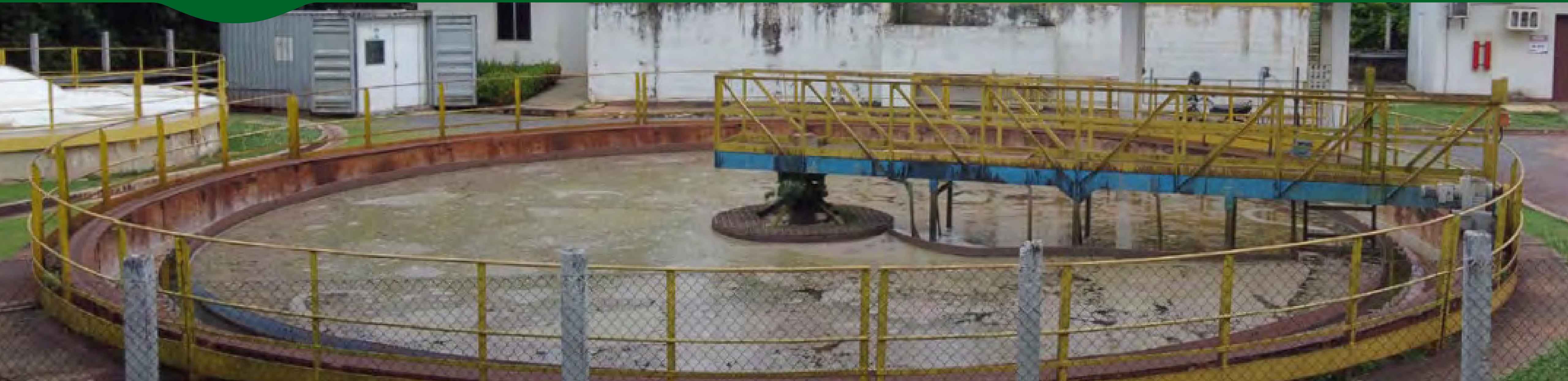
Water Treatment Plant (WTP)
